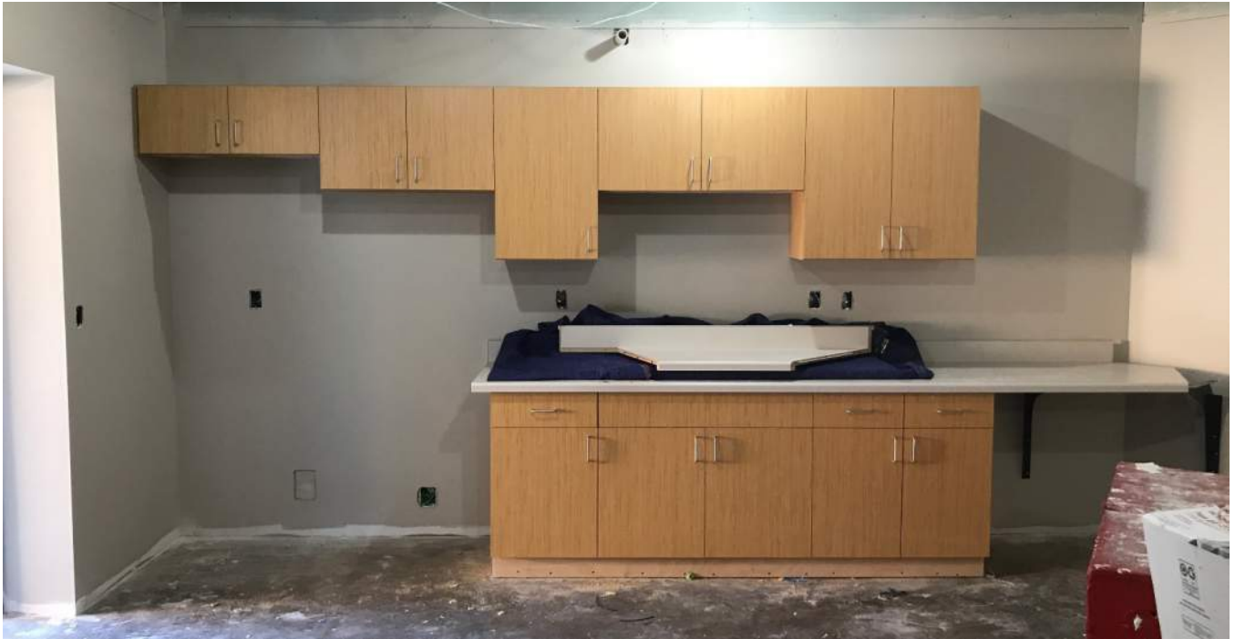
Shown above is some of the casework that has been installed in the new conference room! This space has been completely transformed!
