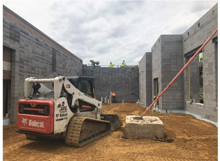
An interior look of the new STEM addition facing West.
