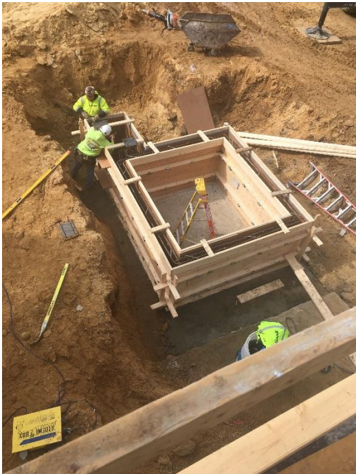
Elevator shaft wall forms!
