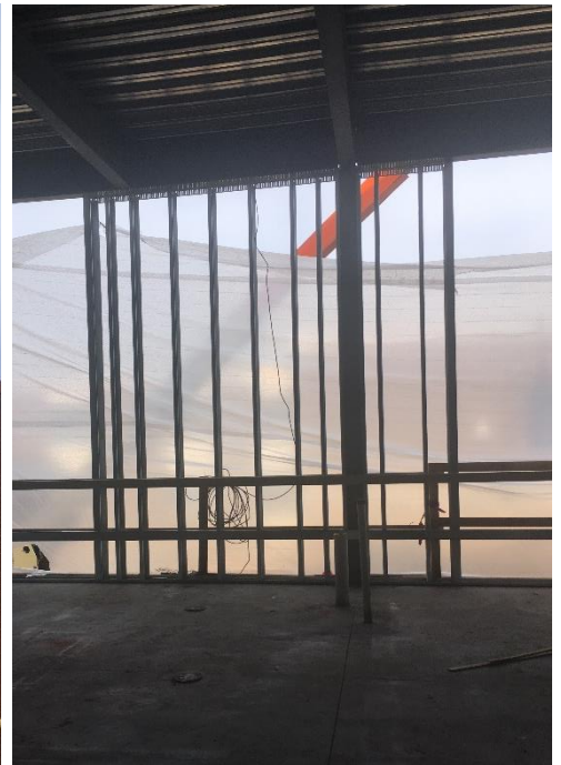
Exterior wall installation!
