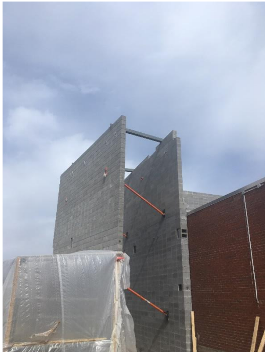
Two story walls up and ready to go!
