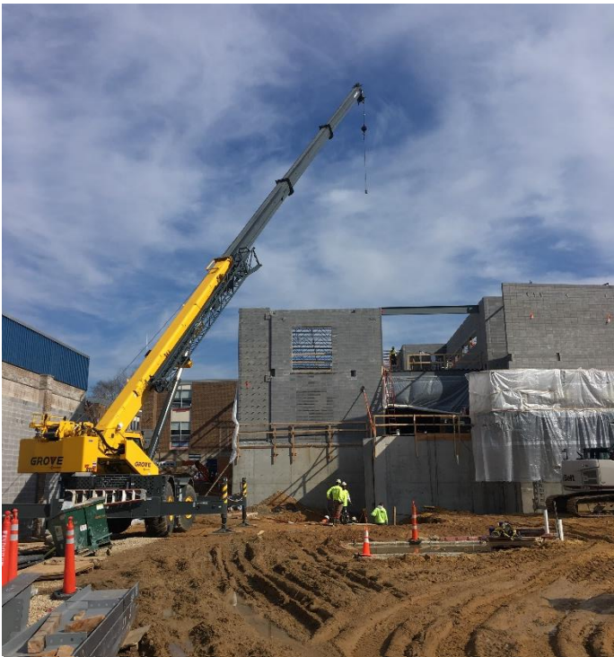
Walls are up in Section C!
