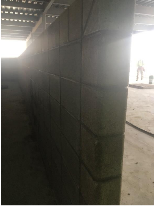
Interior concrete block in the first floor hallway!
