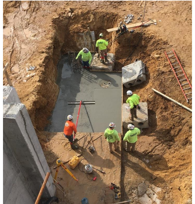
Forming concrete for the elevator Shaft!
