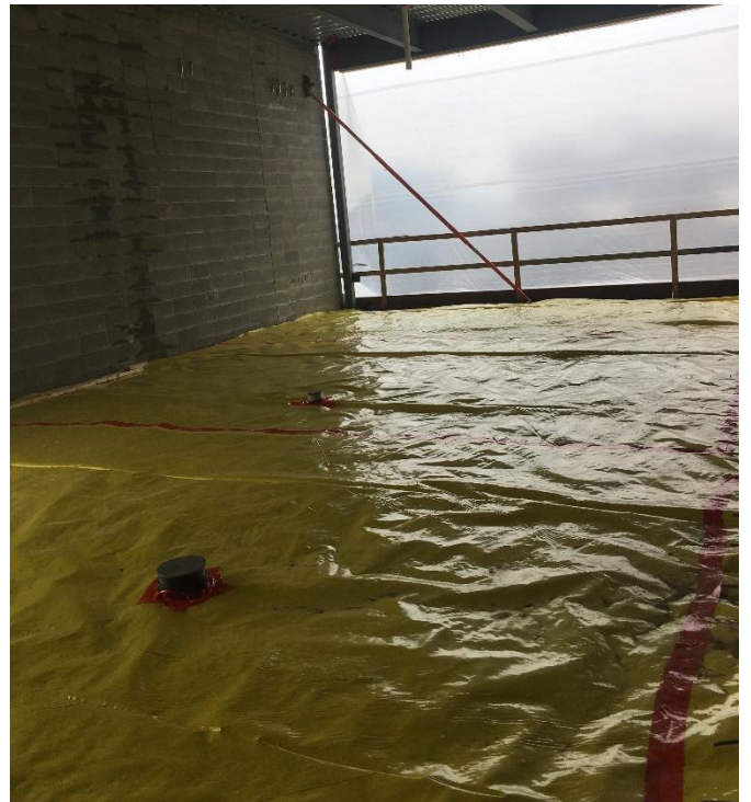
Under-slab vapor barrier set and ready for concrete!
