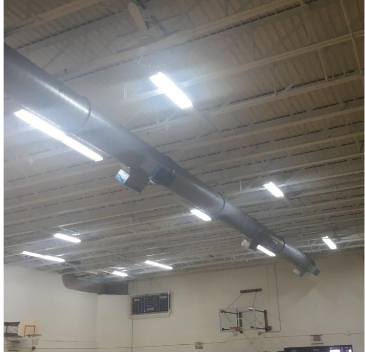
Brand new ductwork in the small gym!
