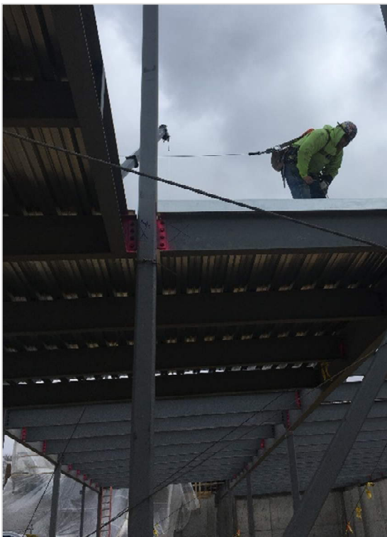
Metal Decking well underway in Section D!
