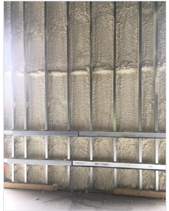
Interior Spray foam is in Section C!
