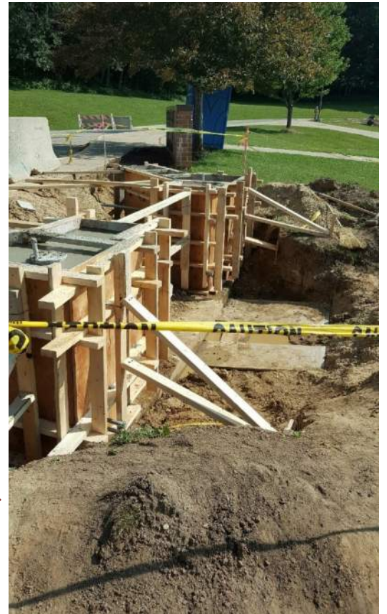
On the right we have a picture of the impressive formwork that was used to form the foundation walls at the new main entry feature for the High School!
