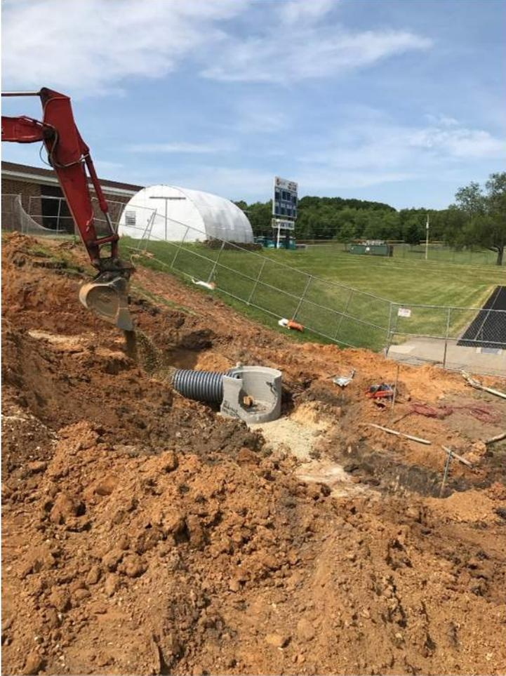
*A view of the underground storm line that was re-routed around the footprint of the new addition.*
