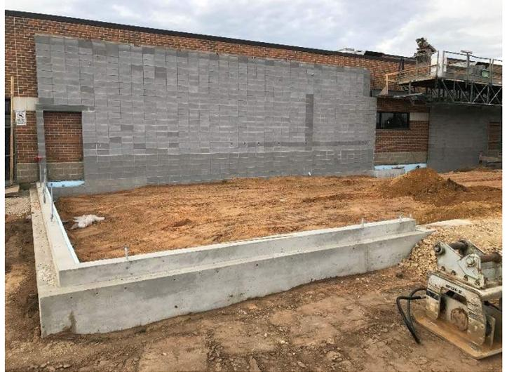
*A look at the progress on the North end addition. This view shows the new CMU fire wall that will lay in between the new and existing STEM areas*
